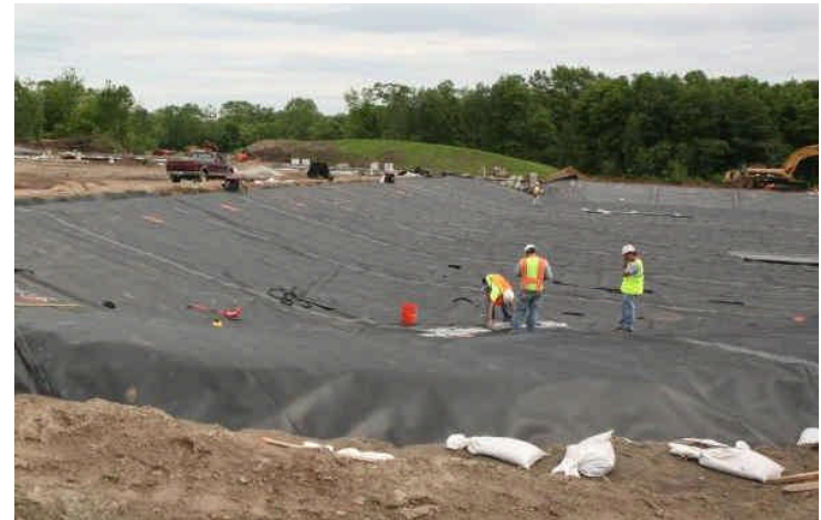
Constructing staging area for sediment.
